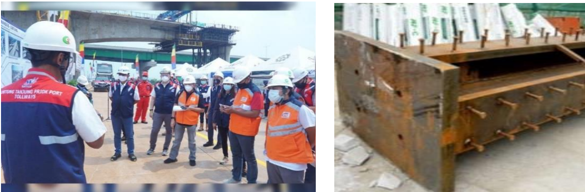
Figure 1. Implementation of construction work during a pandemic (implementing Health protocols and using composite structures)
