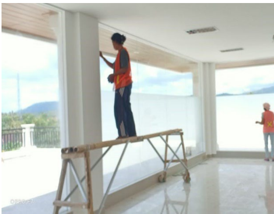
Figure 3: Room Cleaning Work
