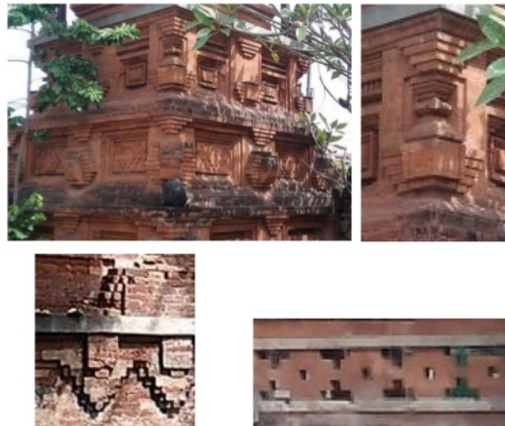
Figure 1. Several forms of pepalihan bebadungan in Denpasar Source: Personal documentation, 2018
