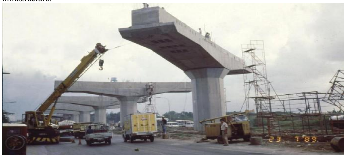
Image 1. Construction of Physical Infrastructure Flyovers
