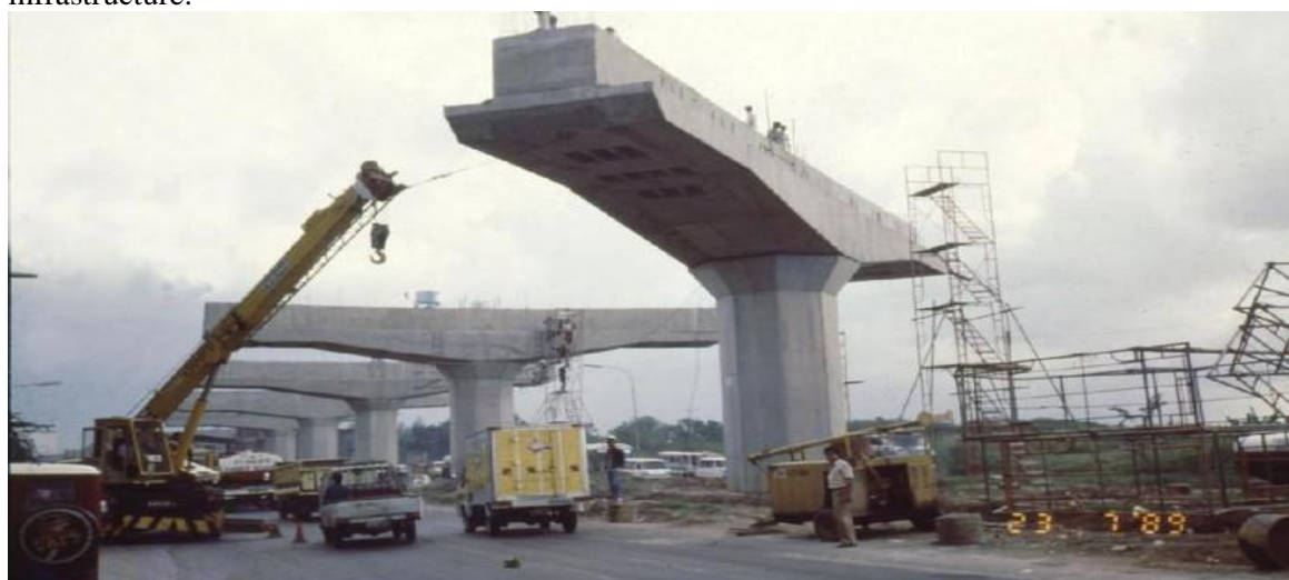
Image 1. Construction of Physical Infrastructure Flyovers
