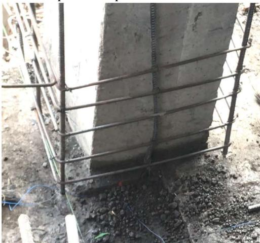
**Gambar. 1** Proses Jacketing kolom
