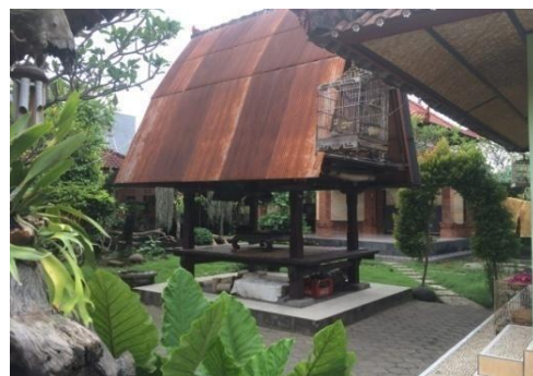
Picture 15 : Jineng in Bali's house Source: Documentation 2019
